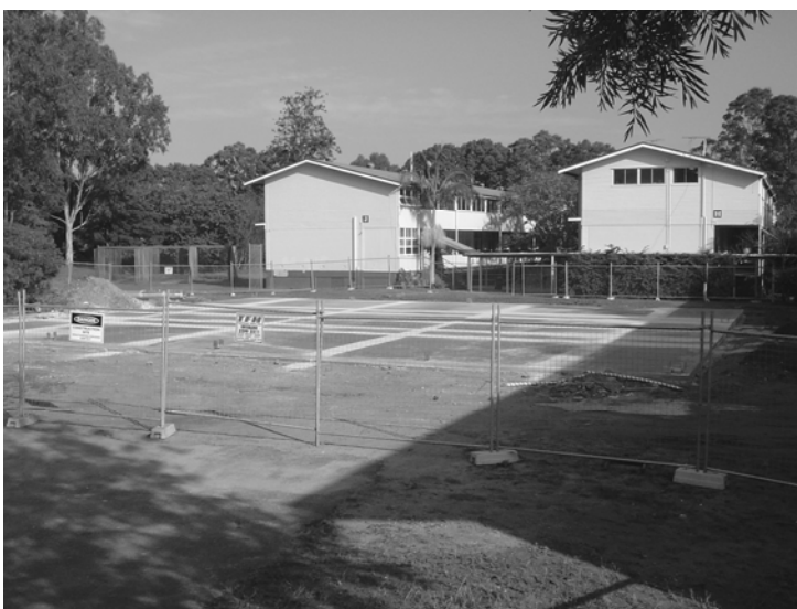
The Sports Shed takes shape
