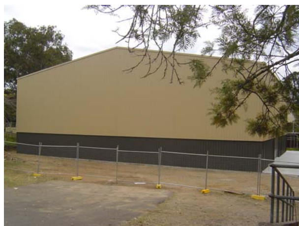
The completed shed
